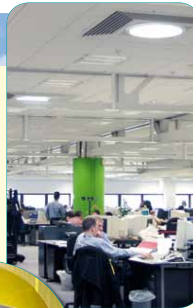
Suncatcher installations at the BMW head offices
